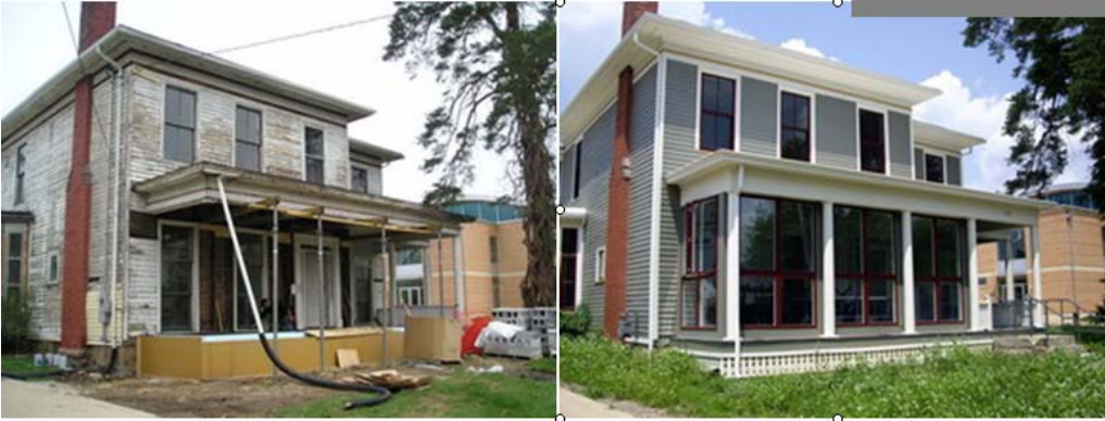
Figure 1. Environmental Studies Laboratory with sunroom before and after renovation
