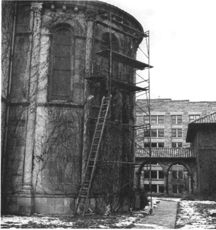
Workmen from John W. Winterich Co. of Cleveland installing stained glass windows designed by Henry Lee Willett in chancel of Fairchild Chapel. 1959
