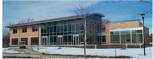
Figure 2. A south-eastern view of the building showing the on-site waste processing system (on right), atrium (center) and 1st and 2nd floor classroom windows (left).
