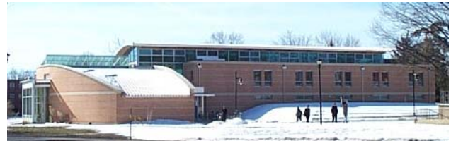
Figure 3. A north view of the building showing the auditorium (left), 2nd floor office windows, and upper windows that light the 2nd floor hallway.
