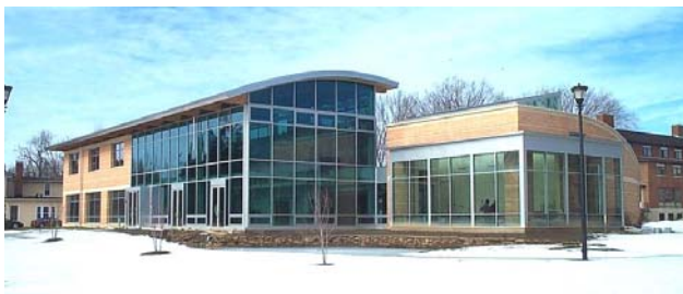
Fig 1. View of the south and east sides of the Lewis Center . PV array is installed on the main, curved roof.
