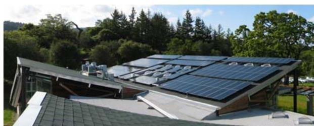
Fig. 1 Photograph of the roof of the west wing of the Sun Field Station. The roof has an inverted geometry with a single central valley for water collection. PV modules are installed on the north part of the roof.
